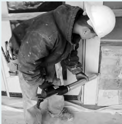
photo provided by: United Professional Caulking & Restoration, Inc.
